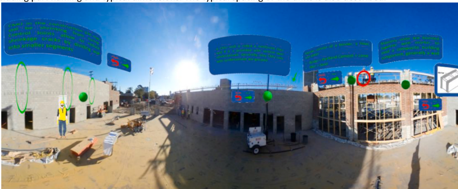
Scene Location 2: Students are shown the composition and use of masonry mortar to construct walls. Additionally, the use of wall reinforcement, grounding, and control joints is defined.
