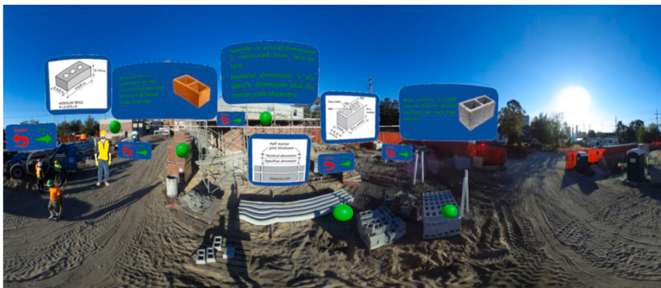
Scene Location 1: Students are introduced to masonry construction. Concrete and masonry units are defined, including part naming and typical dimensions. The typical spacing of the units is also described.
