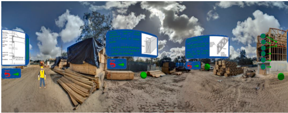
Scene Location 1: Students are introduced to wood platform framing construction. The properties and uses of lumber and truss and the typical composition of a platform framing structure are defined.
