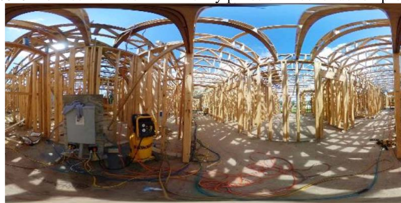
Scene #4: Electrical work in a completed construction project
