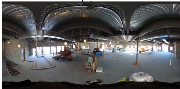
Scene #5: Electrical work and construction safety
