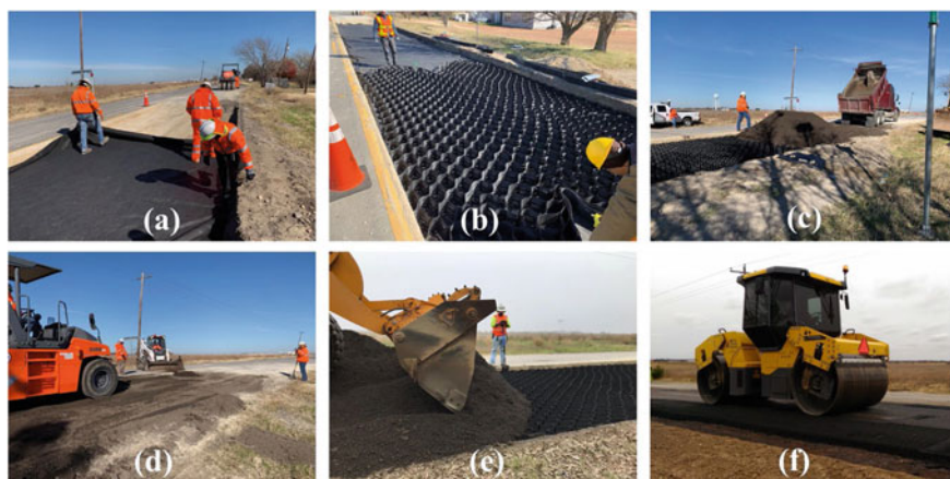
Fig. 2 Construction sequence: a placement of geotextile, b placement of first geocell layer, c placement of RAP, d compaction of GRRB layer, e placement of second geocell layer, and f final surface layer
