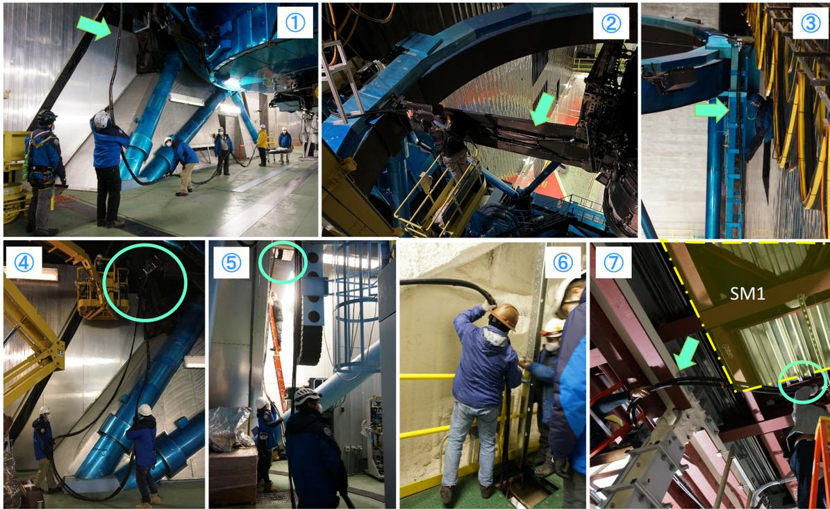
Figure 2. Snapshots of Cable B1 installation process.
