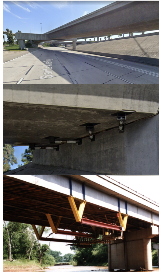
Figure 2: Top: Perspective view of a highway bridge equipped with dampers in Orange County, California, and close-up to the installed dampers (Source: Google Street View 33°51'27.5"N 117°58'46.9"W). Bottom: Highway bridge in Oklahoma, US, instrumented with semi-active variable friction control devices (Source: DoT [69]).
