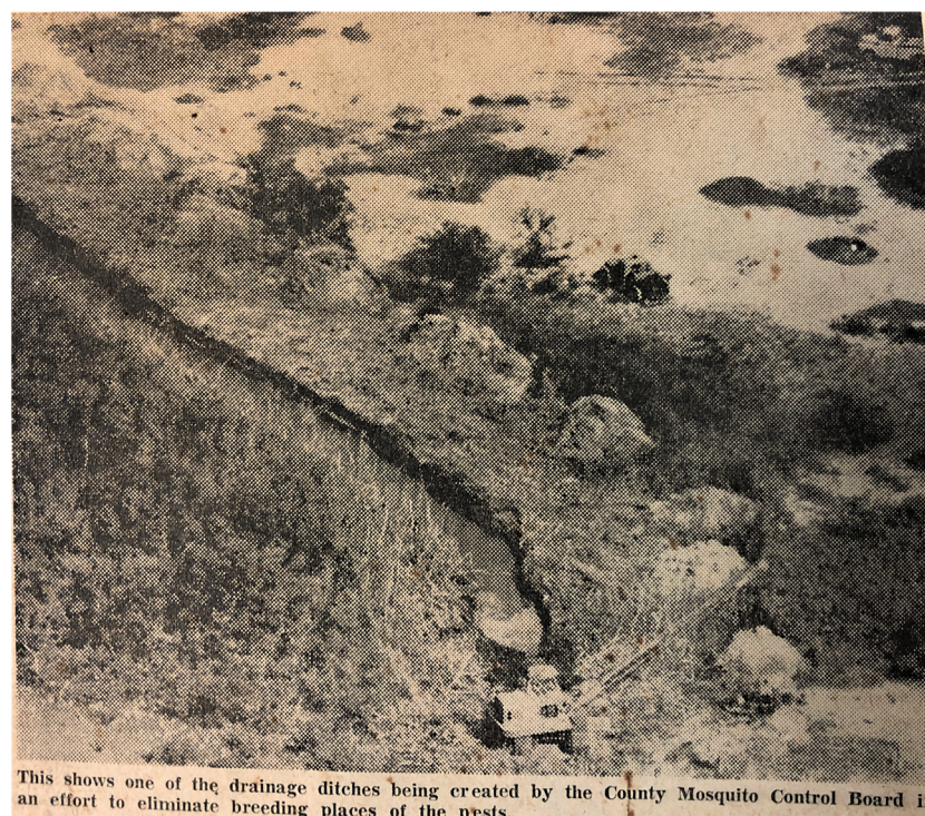
Fig. 14. Dragline operation excavating a linear mosquito-ditch in Pinellas County, Florida, ca. 1956. Clip from Tampa Sunday Tribune, February 2nd 1956.
