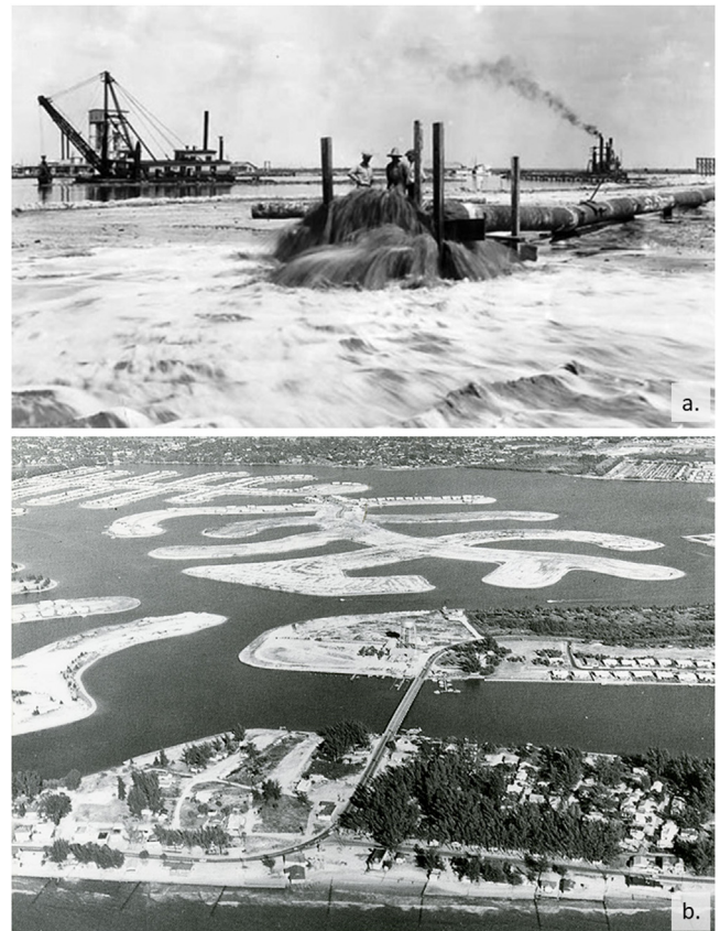
Fig. 2. (a) Dredge operations in the construction of Davis Islands at the mouth of the Hillsborough River, Tampa Bay, ca. 1924. Photo by Bergert Brothers via USF Digital Collections. (b) Dredged landforms and residential construction in Boca Ciega, Tampa Bay, ca. 1950s. Photo via Pinellas County Heritage Village archives.
