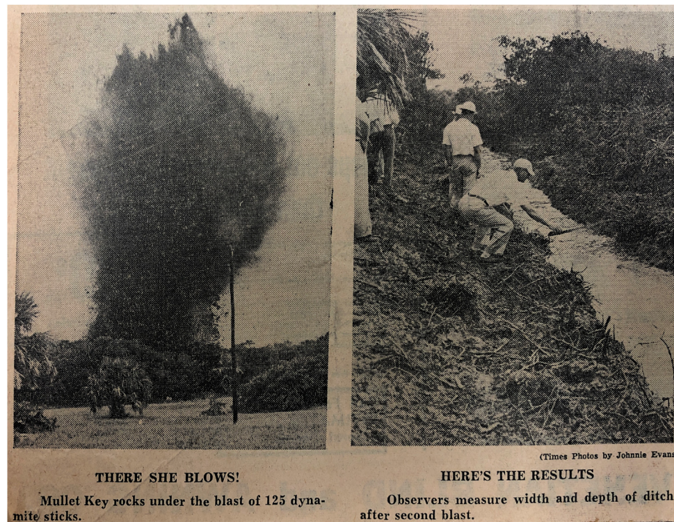
Fig. 13. Dynamite-excavation of mosquito control ditches on Mullet Key, Tampa Bay, ca. 1956. Clip from St. Petersburg Times, June 8th, 1956.
