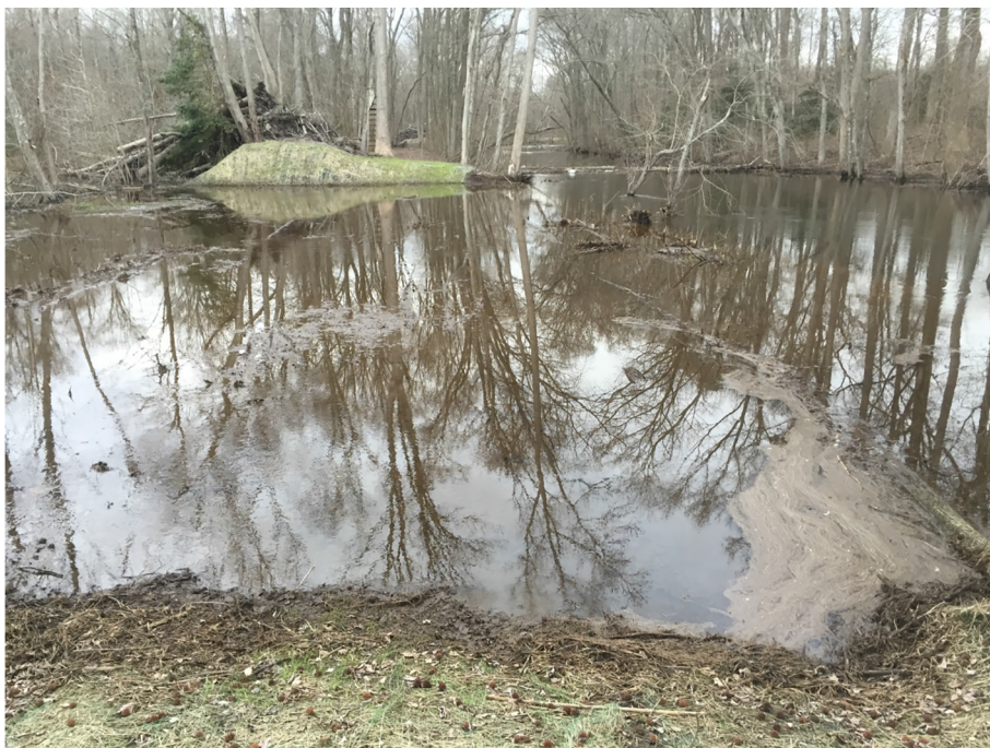
Appendix Photo 2. A levee breach at the restored mainstem site during a flood. Water from the river channel (right) flows across the breach (middle) into the floodplain (left). View is looking across from one end of the breach to the other where the spoil levee continues upstream. Photo taken 8 February 2016. Credit: G. NOE, USGS.
