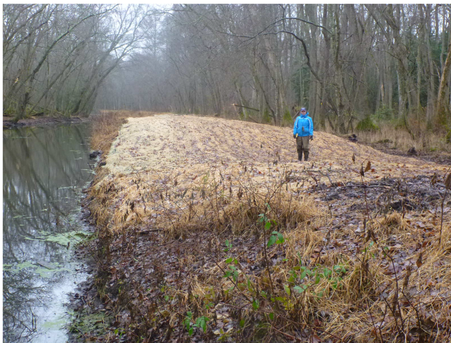
Appendix Photo 1. A levee breach at the restored headwater site during a low discharge period. Water from the river channel (left) flows across the breach (middle, with person standing in low spot) into the floodplain (right) during floods. Photo taken 2 December 2014. Credit: G. NOE, USGS.
