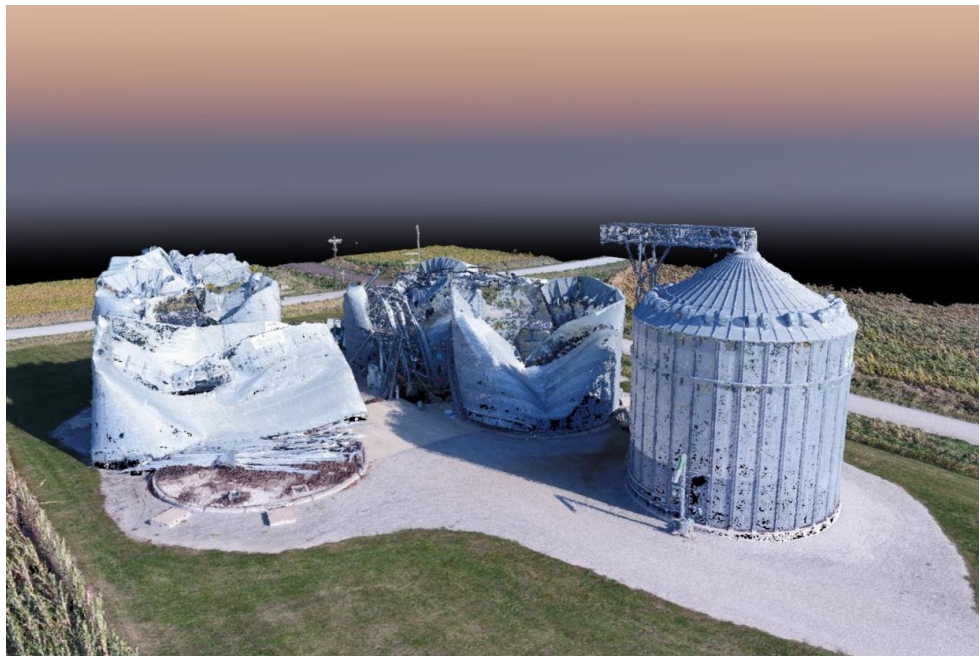
Figure 6. Isometric view of the three-dimensional point cloud of the grain bin site.
