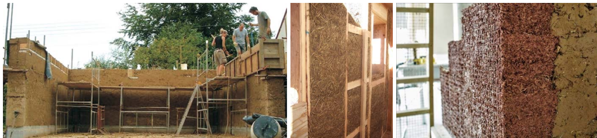
Figure 2: Cob structure made with formwork also known as shuttered-cob, light straw clay wall construction, and a clay-fiber composite.
