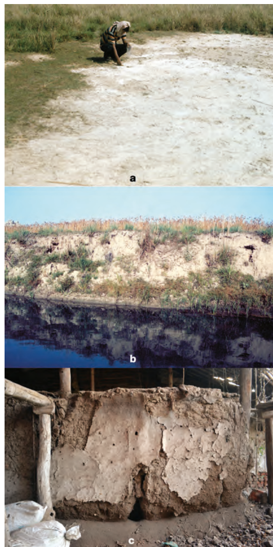
FIG. 12. (a) Reh exposed on the right bank of the Ami River; (b) raw materials on section of the Ami River after the flood recedes; (c) fallen plaster. (Photos: Alok Kanungo)
