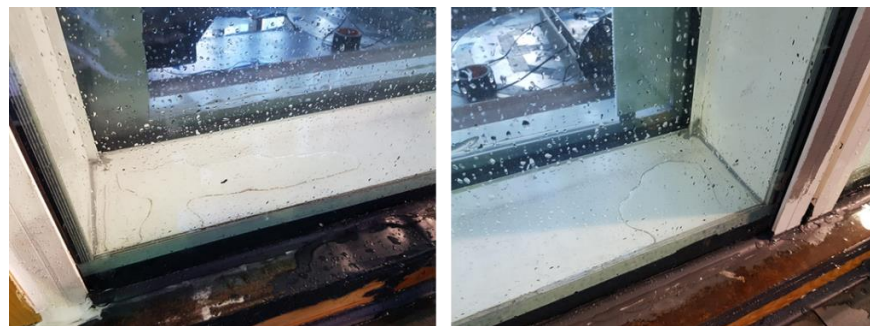
Figure 13. Water penetration in the cavity (Courtesy of WOW Research Team)
