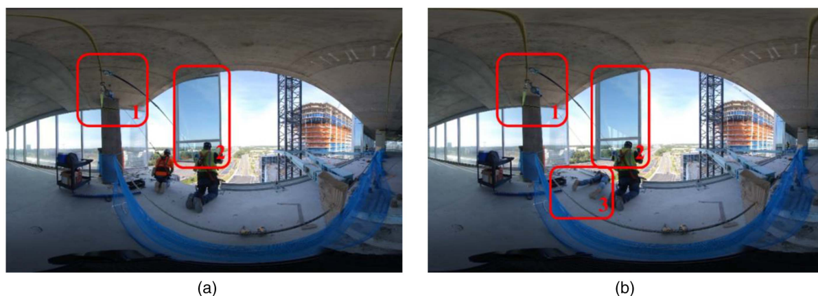
Fig. 1. Example of 360° video scenario, including three dynamic hazards: (a) captured at 5 s; and (b) captured at 20 s. The markings illustrate: 1 = fall hazard; 2 = struck-by hazard; and 3 = fall hazard (Note: images were cropped to magnify focused area).
