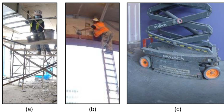
Fig. 8. Example of target and context cues captured from 360 video-based scenarios: (a) tossing material off the scaffold (Struck by Hazard/Target cue); (b) reaching out of the side of the plane (Fall Hazard/Target cue); and (c) tape marking (Struck-by Hazard/Context cue).
