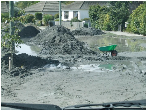
Fig. 1. Picture of post-liquefaction damage in Christchurch, New Zealand, as a result of the 2010–2011 Canterbury Earthquake Sequence. (Photo courtesy of Dr. Lukas Hogan, University of Auckland).
