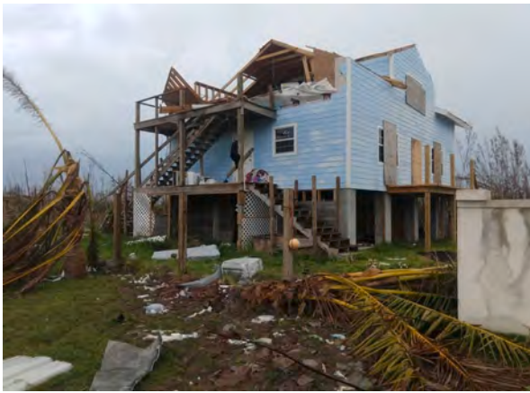
Fig. 1. A post-hurricane survey photo of a one-story elevated house located in Abaco Island shows the wall and roof damage caused by hurricane Dorian in 2019 [1].
