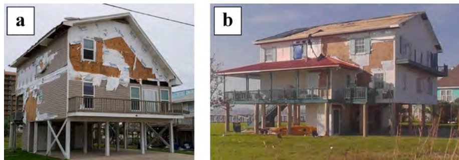
Fig. 2. Post-hurricane survey photos of two-story elevated houses which sustained wall and roof cladding damage in 2020 (a) Hurricane Sally, and (b) Hurricane Laura [1].
