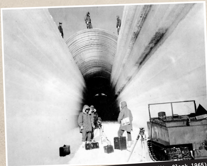
Figure 6: Roofing a finished trench (image credit: Clark 1965).
