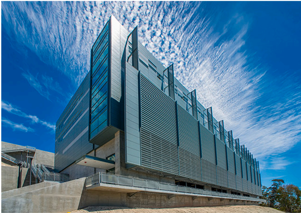
Fig. 7. Building 59 at LBNL, Berkeley, California.
