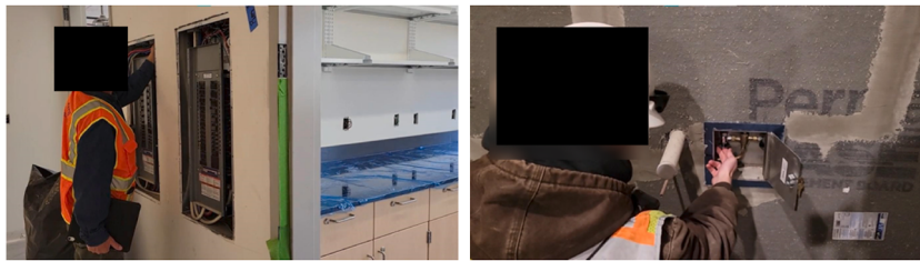
Fig. 8. Examples of contact-based inspection. Left: the inspector checks the electrical wires for proper connection. Right: the inspector checks the connection of valves through a plumbing access panel.
