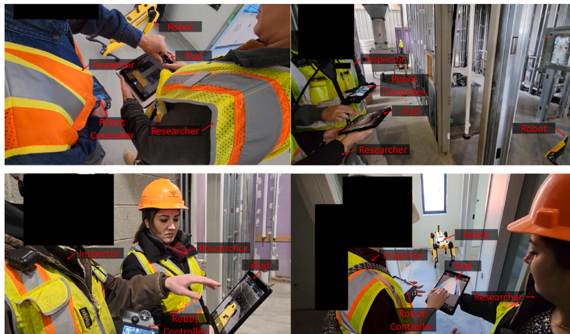
Fig. 3. Site inspectors performing virtual inspection using a quadruped robot and ipad with video stream of the robot-mounted camera.
