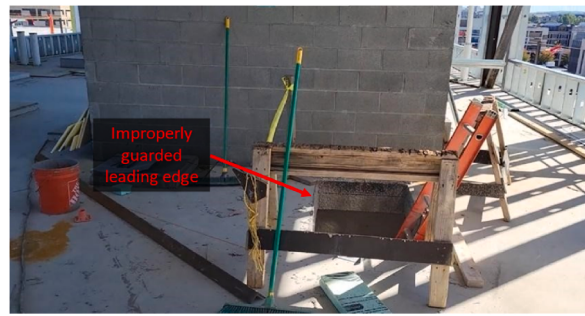
Fig. 10. An improperly guarded leading edge causing a potential safety hazard.
