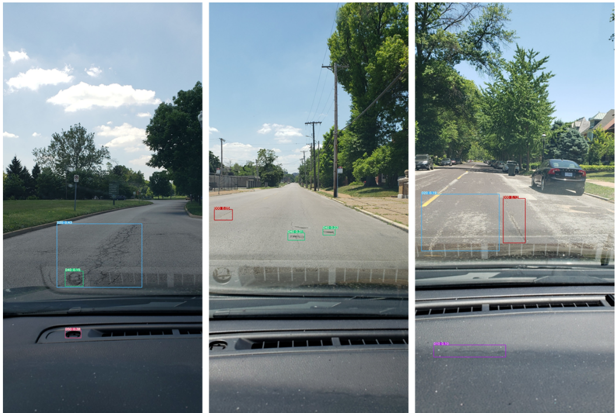
Figure 10: Pavement. distresses detected from video data
