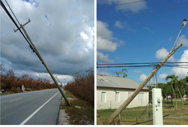
Fig. 2. Sample images of damaged utility poles from the gathered dataset. [35]
