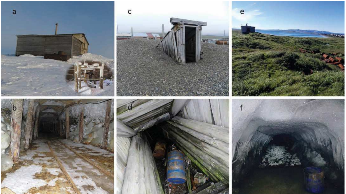
FIG. 6. Siberian cellars: a) ventilation shafts in Lorino, Chukotka, b) Lorino horizontal cellar with rail, c) wooden old Russian style cellar with double ventilation, d) inside a cellar at Uelen abandoned due to flooding, e) entrance shed of Inchoun cellar on polygonal ground, and f) inside of Inchoun cellar before flooding in 2016.
