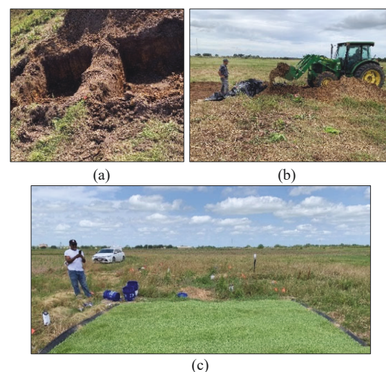
Fig. 1. (a) excavation of the test pits (b) soil backfilling after a 6-mil plastic sheet placed on the bottom of the excavation floor and inside the side wall of excavated pits (c) textured geomembrane layer placed over the smoothen compacted layer overlain by engineered turf
