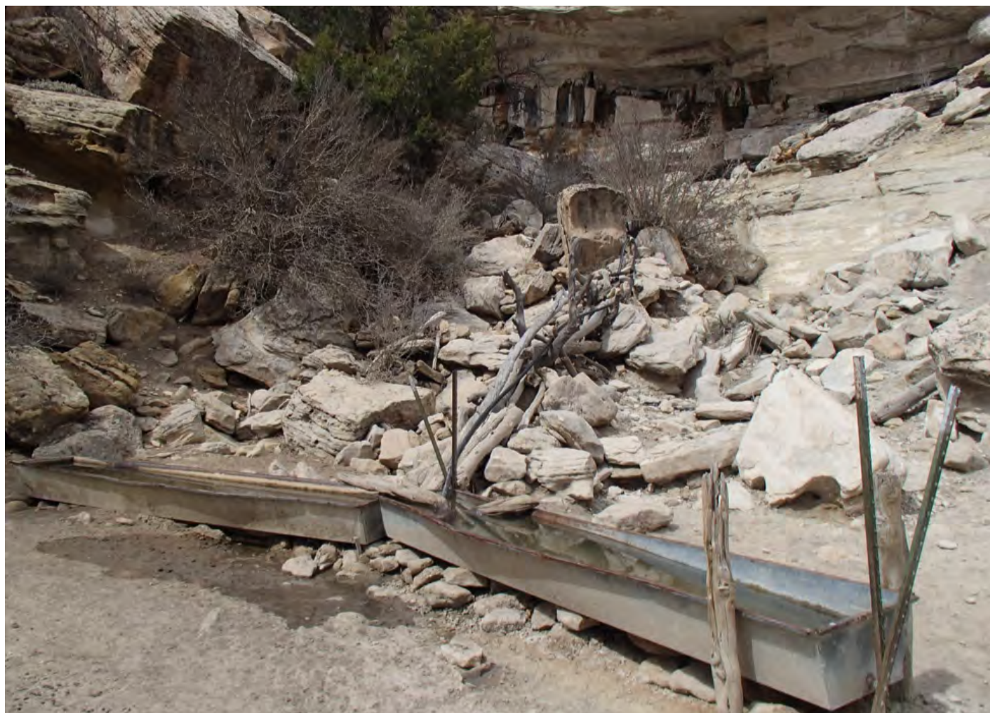
At Waterfall Spring, an unregulated water source on the Navajo Nation, water is collected and funneled to watering troughs downhill of a spring. Source: Joseph H. Hoover.
