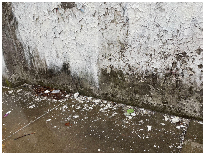
Figure 3. Sidewalks are littered with paint chips from dilapidated viaducts
