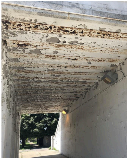
Figure 2. Decaying paint peels from the walls and ceilings of viaducts
