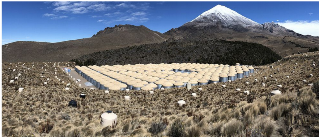
Fig. 1. The HAWC observatory, seen looking north from the Sierra Negra volcano. The Citlaltepetl volcano is visible in the background. The primary detector (HAWC) is at the center, surrounded by the smaller plastic tanks (outriggers) not discussed in this paper (see Section 7). Credit: The HAWC Collaboration.
