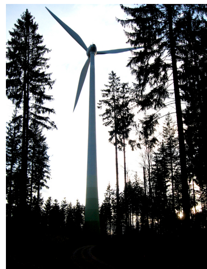
Figure 1. A wind turbine located in a forest in southwestern Germany.
