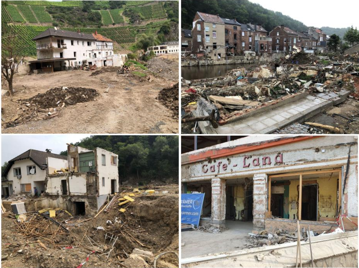
Figures 2 a-d: Observed building damage in various locations. a (Top Left): Walporzheim, Germany (Lat: 50.53245, Lon: 7.06271); b (Top Right): Pepinster, Belgium (Lat: 50.56925, Lon: 5.80531); c (Bottom left): Walporzheim, Germany (Lat: 50.53264, Lon: 7.06146), d (Bottom right): Altenahr, Germany (Lat: 50.516144, Lon: 6.988238)
