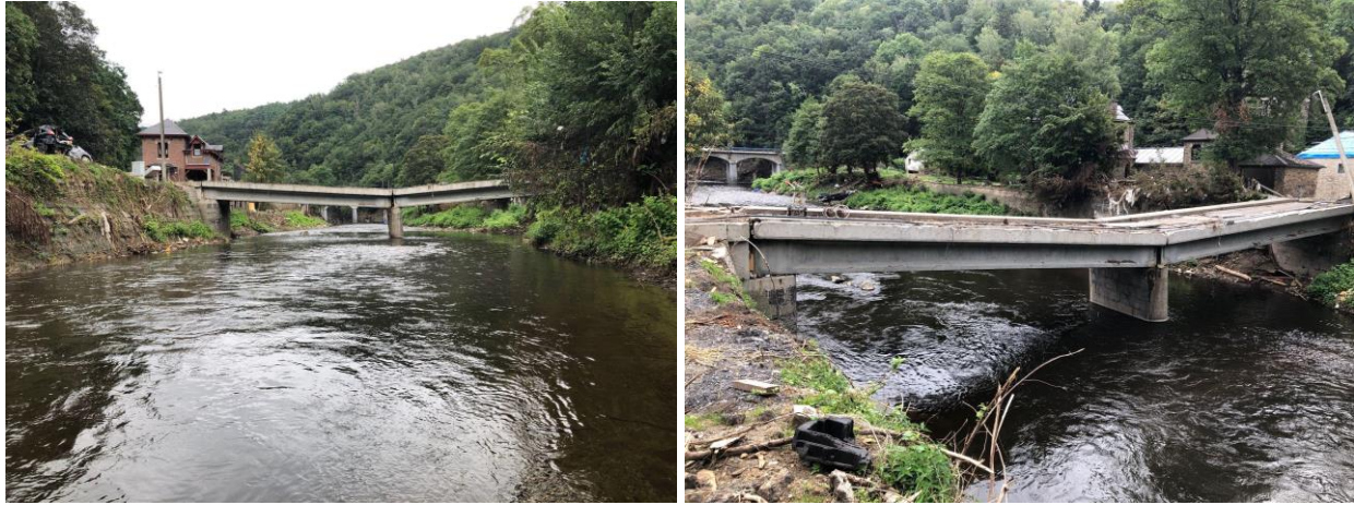
Figure 4 a-b: Ry Fenderie bridge in Trooz, Belgium. Photographs taken via mobile phone. (Lat: 50.57080 Lon: 5.68953)
