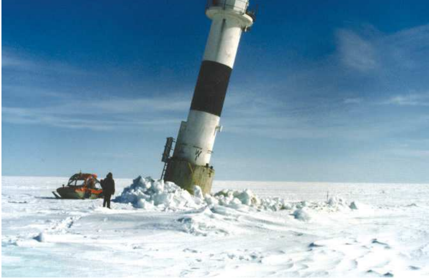
FIGURE 2. THIS LIGHTHOUSE in the Baltic Sea was photographed after it interacted with the wind-driven ice cover. (Adapted from ref. 18.)
