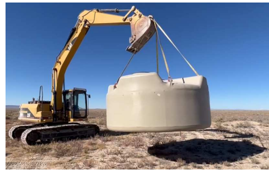
Figure 5: Auger@TA station being put in place at its deployment site with an excavator.
