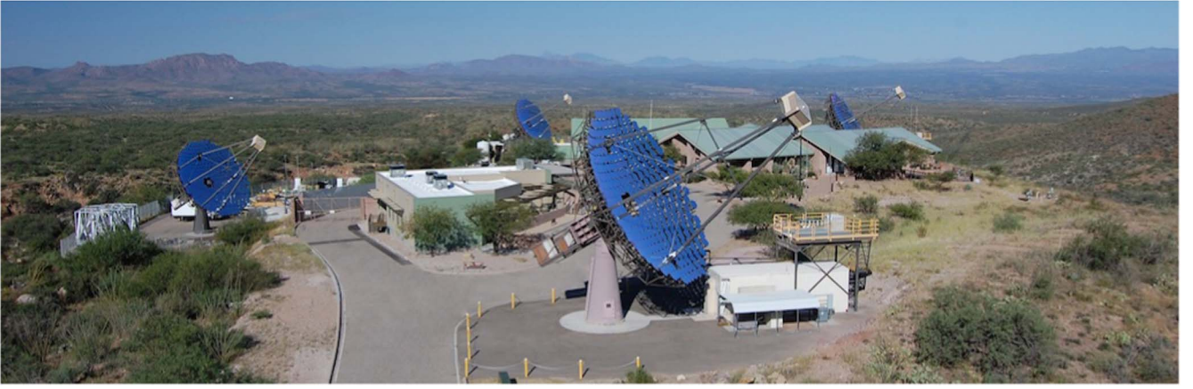
Figure 1. Elevated view of the VERITAS array located at the base of Mount Hopkins near Tucson, AZ. Pictured are the four individual telescopes, which are roughly 100 m apart, the Fred Lawrence Whipple Observatory visitor center, and the VERITAS control building (with the white roof). Image from Abeysekara et al. (2016).
