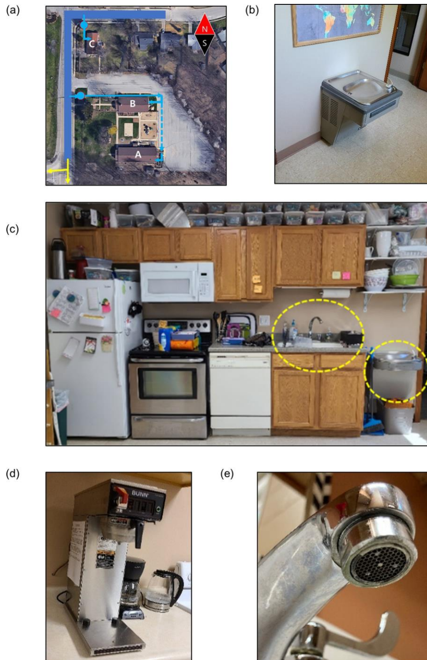
Fig 1. (a) Site property with building A, B and C with estimated location of public water supply pipe (blue), two water meters (sky blue circle) and service line to each building (sky blue) and where splits to deliver to building A (dotted sky blue), (b) Elkay drinking water fountains installed for kids' height, (c) all classrooms had their own sinks, drinking water fountain, and appliances, (d) coffee maker connected to the plumbing in building A, and (e) particulates in the aerator before removal.
