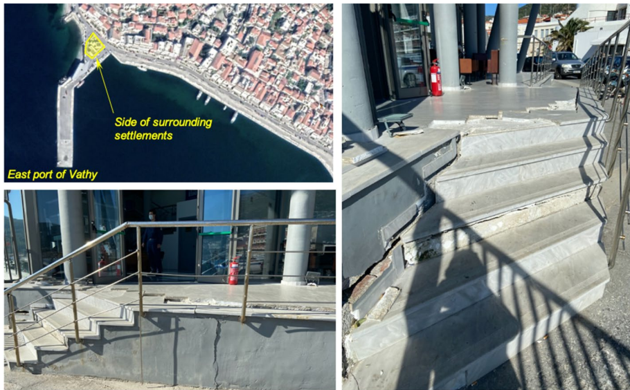
Fig. 4 Damage observed around the Port authority building in Vathy, Samos (location: 37^{\circ}45'27.0'' N 26^{\circ}58'15.4'' E). The cracks indicate soil settlement/distortion around the building which remained intact and functioning 8 days after the earthquake
