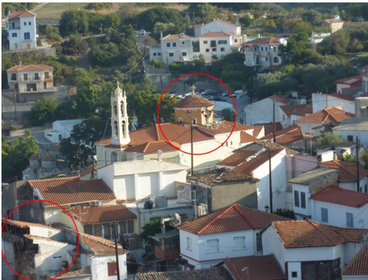
Fig. 26 Ano Vathy: Close view of the damaged dome of the Church of Metamorphosi Sotiros and neighboring building. (Photo by Christos Giarlelis, HAEE/ETAM Team)
