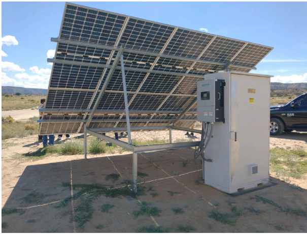
Fig. 1. Image of the Sol-Ark off-grid electrical system. The inverter, charge controller, battery bank and data acquisition system are in the enclosures in the foreground. The bi-facial 3.8 kW PV array tilted at 35 degrees in the background.
