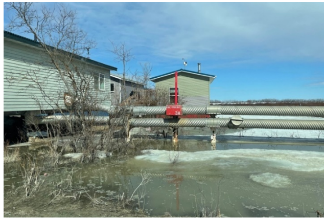
Figure 1: Piped water systems with above-ground pipes due to concerns with tundra freeze and melting causing subsidence
