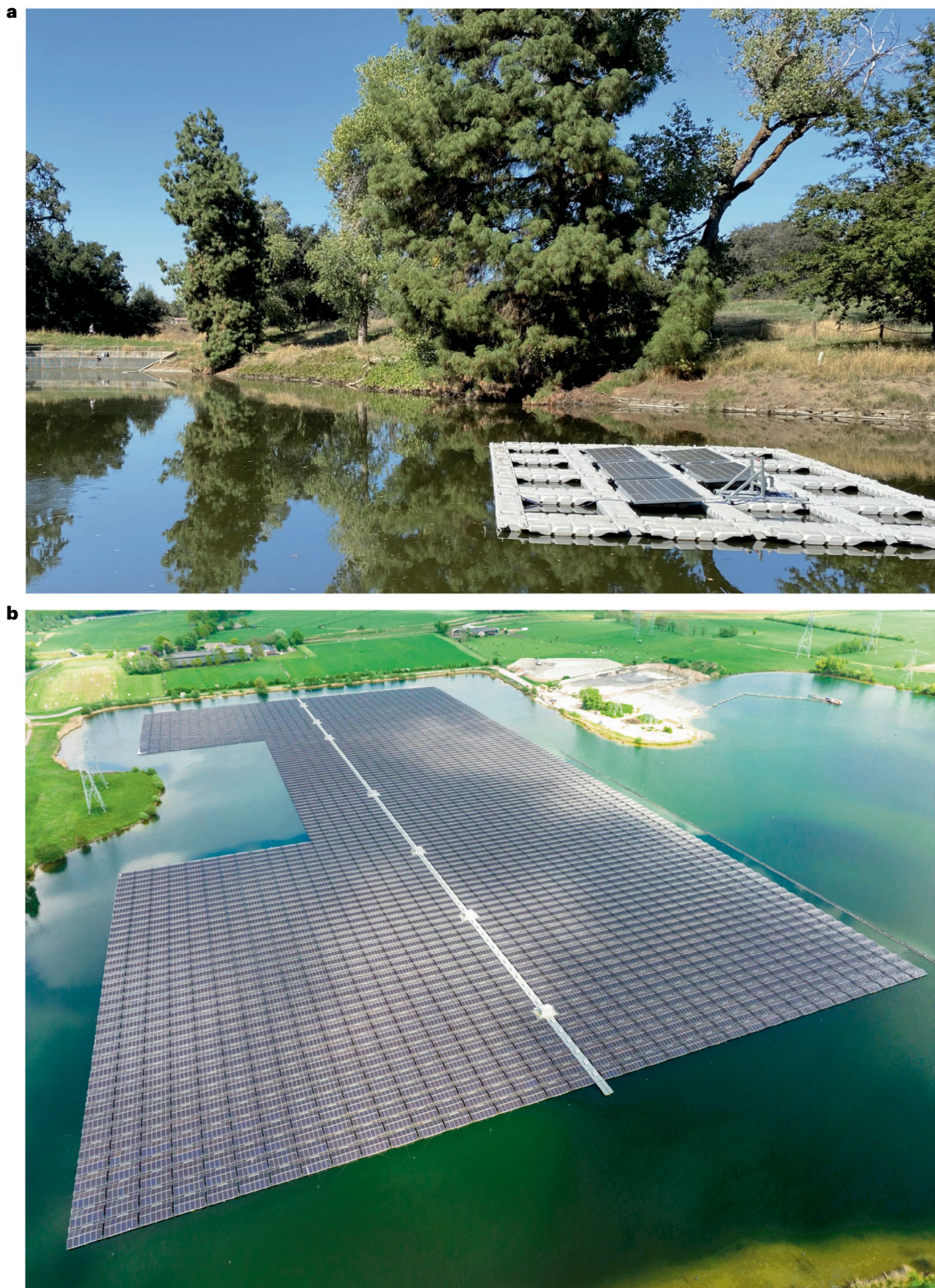
Fig. 3 | Examples of floating photovoltaics. a, A floating photovoltaic system around the University of California at Davis designed to reduce green algae by improving aeration with solar energy. b, A floating solar farm producing clean renewable electricity energy and reducing reservoir evaporation in Flevoland, the Netherlands.
