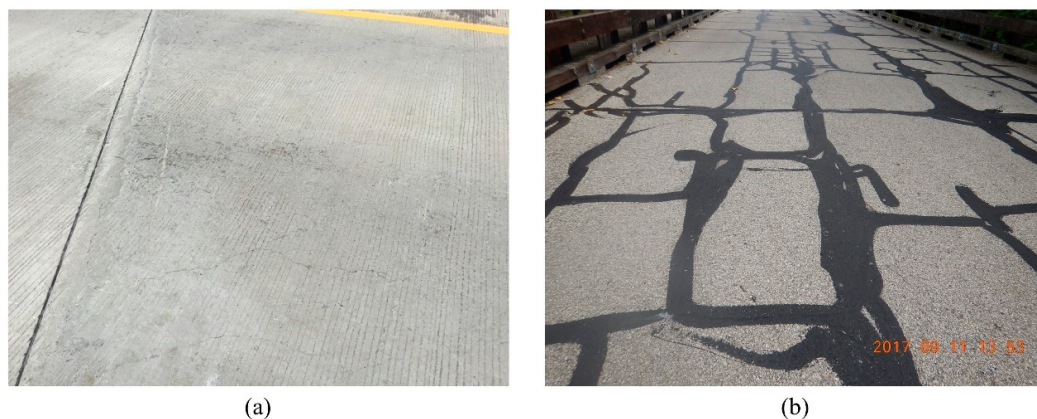
Figure 3. Examples of (a) “non-Sealed” images and (b) “Sealed” images for Image Classifier II.
