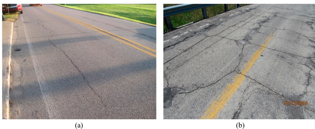
Figure 4. Examples of (a) “Normal Crack” images and (b) “Map Crack” images for Image Classifier III.
