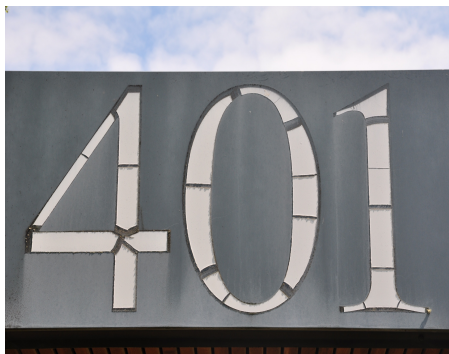
FIG. 2. Cracked lettering at Ecole Polytechnique, Palaiseau, France
