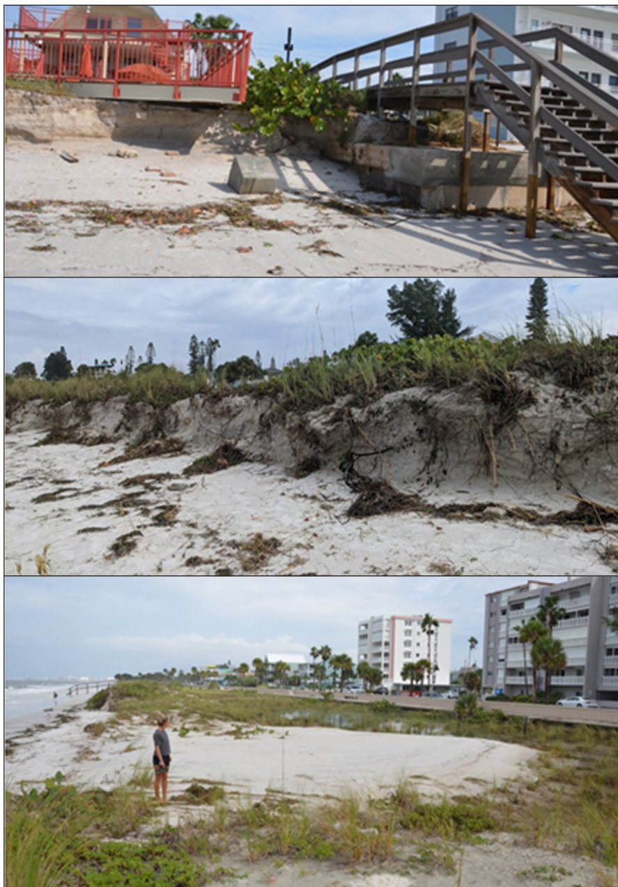
Figure 6. Examples of dune erosion and overwash deposit induced by TS Eta.
