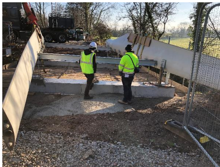
Figure 9. BladeBridge during assembly showing the cradles supporting the blades (prior to installing all the deck beams and plates).
