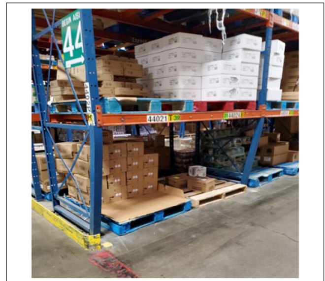
Figure 1. An example of 2-tier racking commonly found in grocery distribution centers.
