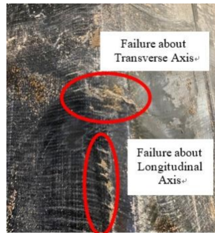
Fig. 26. Sheet pile failure.
