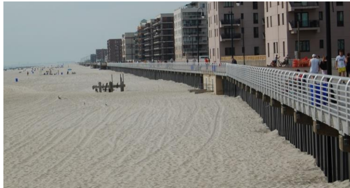
Fig. 1. Sheet piling of Long Beach, New York (Photo courtesy of Creative Composites group).
