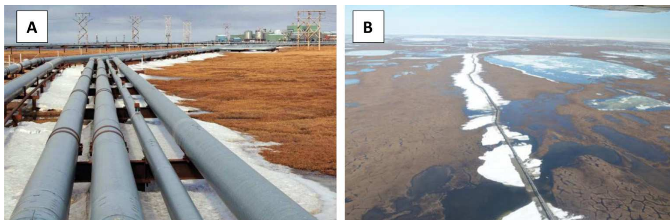
Fig. 16. Photos showing snowmelt patterns for different positions in and around Prudhoe Bay. Photo A (by Martha Raynolds, June 2014, published in Walker et al. 2014) illustrates that many of the pipelines in Fig. 3 are composed of multiple parallel pipes that, in combination with an adjacent access road, create large snow drifts and affect large areas of tundra. Photo B (by Benjamin M. Jones, June 2014) shows a section of the Trans-Alaska Pipeline System and late-melting snowdrifts. This delayed snowmelt along the pipeline is clearly shown in Fig. 4 (yellow lines near the middle of both images).
