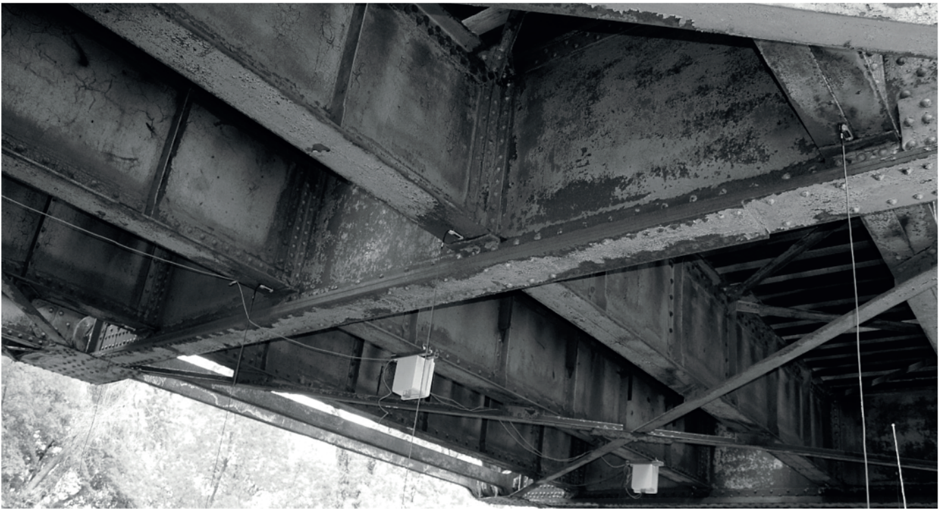
Fig. 4. Partial cross section of stringers and floor beam system with installed strain transducers.
