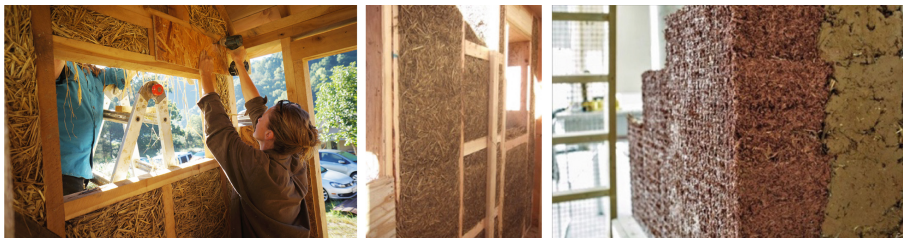
Fig. 2. Light straw clay workshop by The Year of Mud; Light straw clay monolithic wall construction, and; Manually constructed earth-fiber composites. Image sources: (Goodhew et al. 2021; Baker-Laporte, Laporte 2015).
