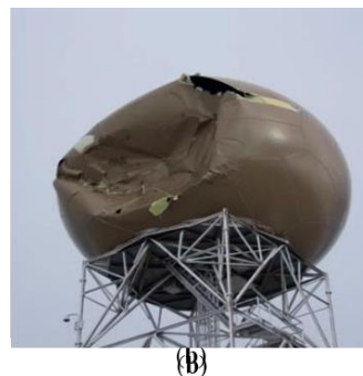
Figure 2. (a) The New Orleans Superdome badly damaged during Hurricane Katrina (by Trahan Architects/Asm Global); (b) The Reno/Virginia peak dome collapsed due to strong wind gusting (by NWS Reno, Nevada).
