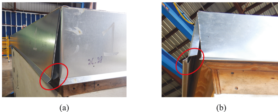
Fig. 21. (a) Configuration 1: premature fascia and cleat disengagement, and (b) Configuration 4: cleat and fascia oscillating together.
