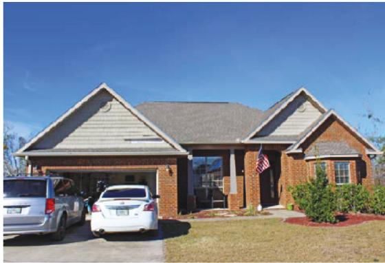
(a) Recently reroofed post-FBC house
