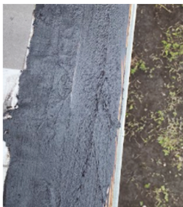
(a) Adhesive extending to the rake edge tip
