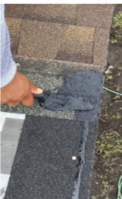
(b) Adhesive over the headlap
