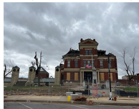
(h) Damage to the Graves County Courthouse: Destroyed
