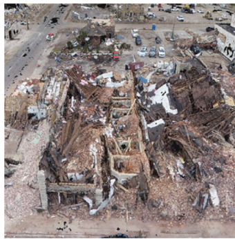
(a) Roof Collapses
