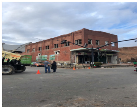
(d) The isolated two-storey structure: Severely Damaged
