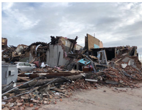
(c) Row Buildings on Broadway: Destroyed
