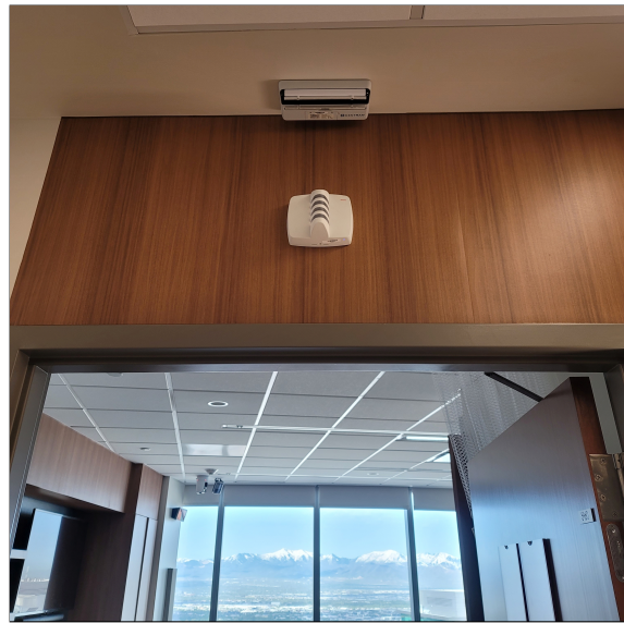
Fig. 3. As part of the smart hospital technology, real-time locating system sensors are installed on the ceiling of the hallways and above the patient doors. These sensors can track the movement of the patients, providers, and equipment throughout the hospital.
