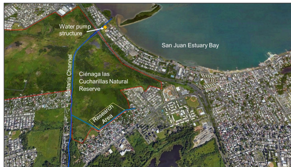
Figure 3. La Malaria flood control channel (represented by blue lines) positioned northwest of the delineated research area (highlighted with a yellow line) at Ciénaga Las Cucharillas Natural Reserve (outlined with a red line). The location of the outflow water pump structure is indicated by a yellow square at the channel's downstream point of discharge.
